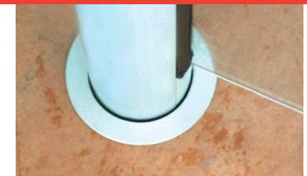
CORE DRILLED
